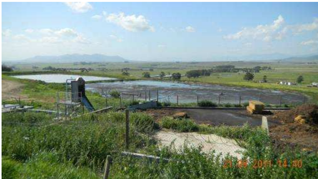
Figure 7: The existing treatment dam at Keibees with separator left in foreground, aerobic dam in the middle and the anaerobic dam to the left at the top.
