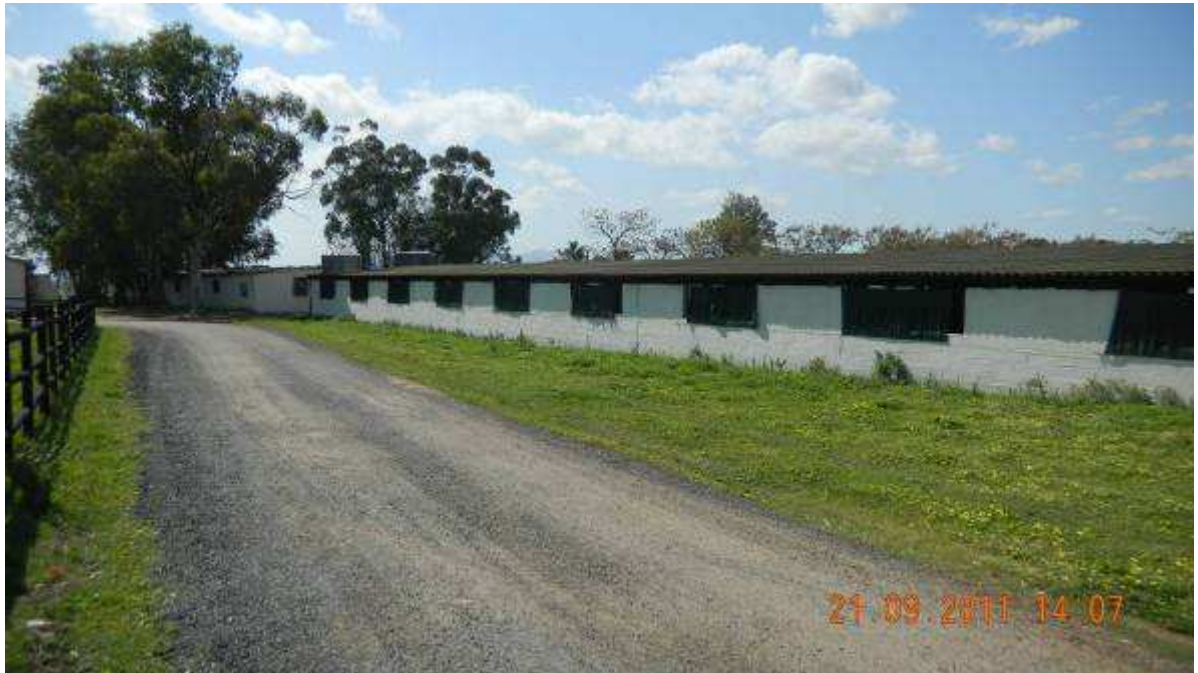
Figure 1: Pig houses at Zandam looking north.
