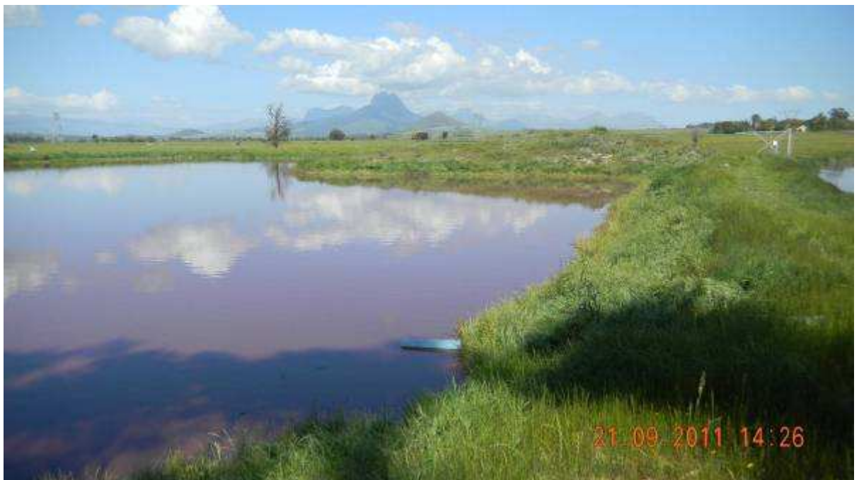
Figure 9: Existing Aerobic Pond at Zandam
