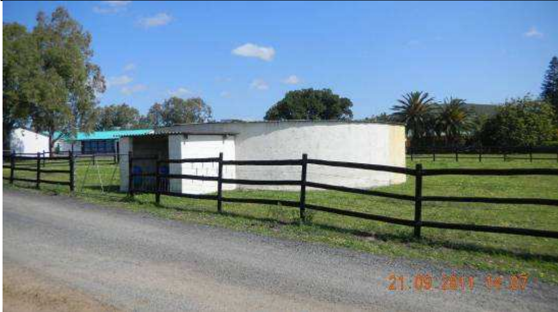
Figure 3: Potable water storage dam at Zandam
