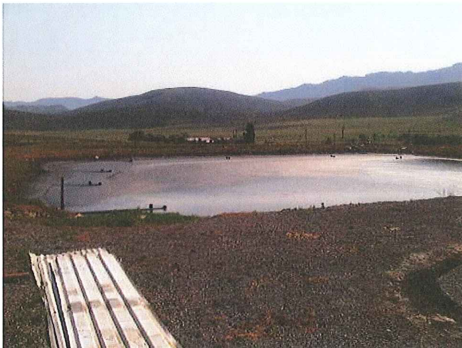
Figure 8: Existing Aerobic Pond
