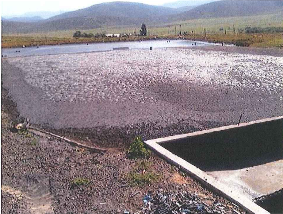
Figure 7: Existing Anaerobic pond.
