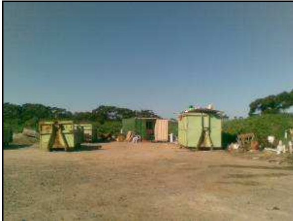
Building rubble storage area.
